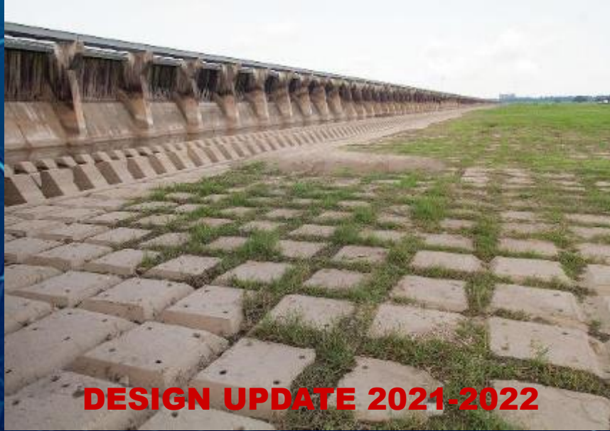
Articulated Concrete Block Mattress Channel Bottom
