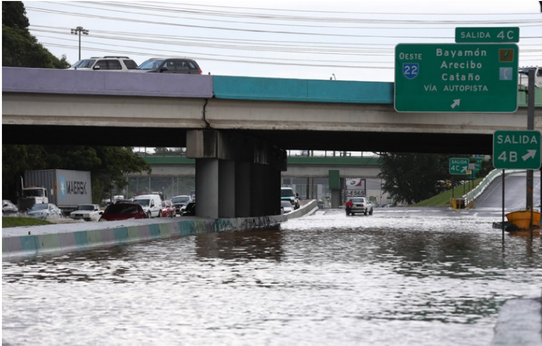
Photograph 7 - Quebrada Margarita Flooding at PR-2 and PR-22
